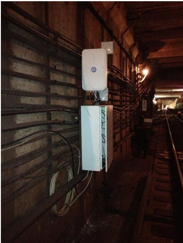
Pic. 3 Stationary point with WiBOX PA D4M5-20HVX MIMO 4x4 directional antenna and Cisco router installed inside.
